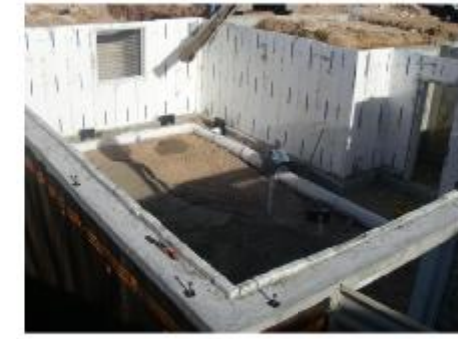
BELOW SLAB DUCTING
